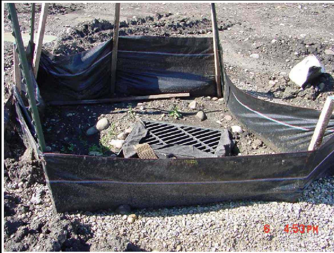
Good Storm Sewer Protection
