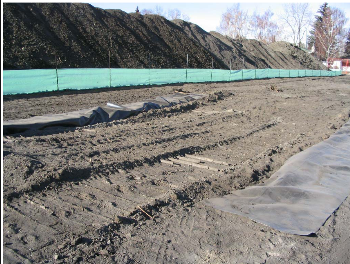
Tarped Fuelling Area
