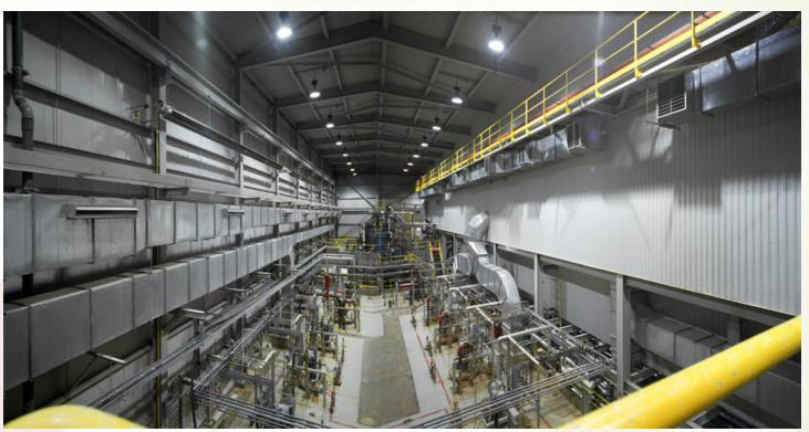
Powerful ventilation system; lead flooring on worker platforms; graded flooring for clean-up ease
